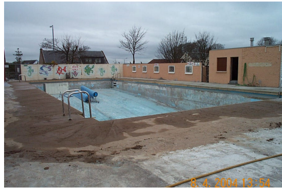
The pool before refurbishment in 2006
