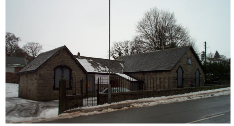
The school prior to the commencement of work
