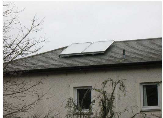
More Solar Panels on Potala House
