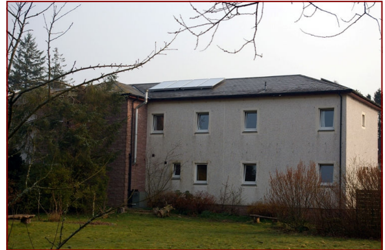
The Solar Panels on Potala House
