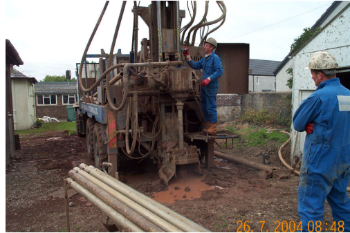
The very long, rotating pneumatic drill at work
