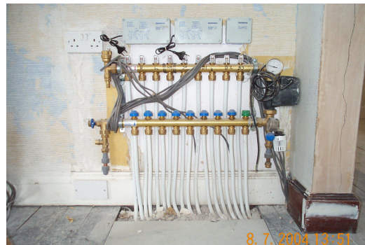
The manifold for up to nine temperature zones
