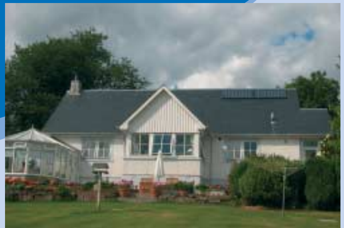
Mr Prior's home was the first home to benefit from an Energy Saving Trust funded solar water heating system.
